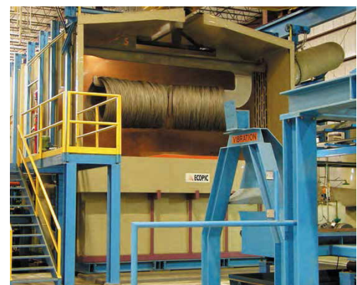
Acid pickling for oxide removal
